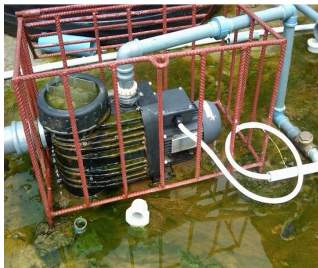
Figure 3: Leaking surface water pump of the solar installation at Ide Village
