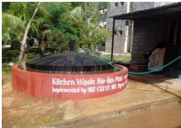
Figure 1: Photograph of 60 kg/day kitchen waste biogas plant at Postal Training Centre, Mysore
