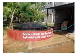
Figure 1: Photograph of 60 kg/day kichen waste biogas plant at Postal Training Centre, Mysore
