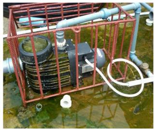
Figure 3: Leaking surface water pump of the solar installation at Ide Village
