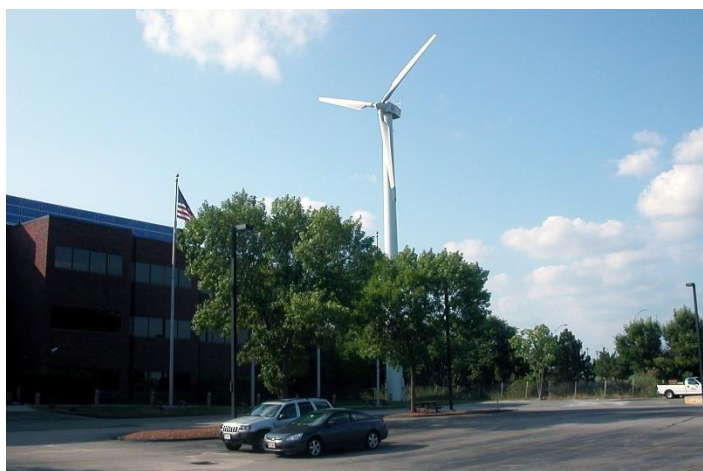
Figure 4. Wind Turbine at the offices of the International Brotherhood of Electrical Workers (100 kW, 21 m blades diameter and 35 m tower). (Massachusetts, US) Source: [27].
