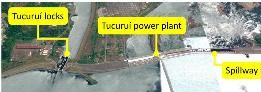
Figure 1. Overview of the Tucuruí hydropower dam and its locks.
