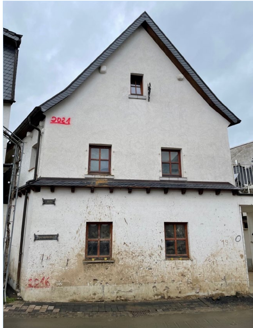
Flood markers at a central building in Dernau indicating the flood levels of 2016, 1910, 1804 and 2021 (bottom to top). Michael Szönyi, 5.4.2022.
