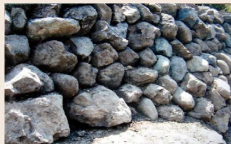
A newly built stone wall (Photo by WV Alangui)
