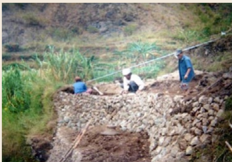
Building a stone wall (Photo by WV Alangui)
