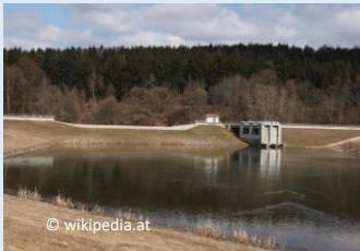
Flood retention basin
