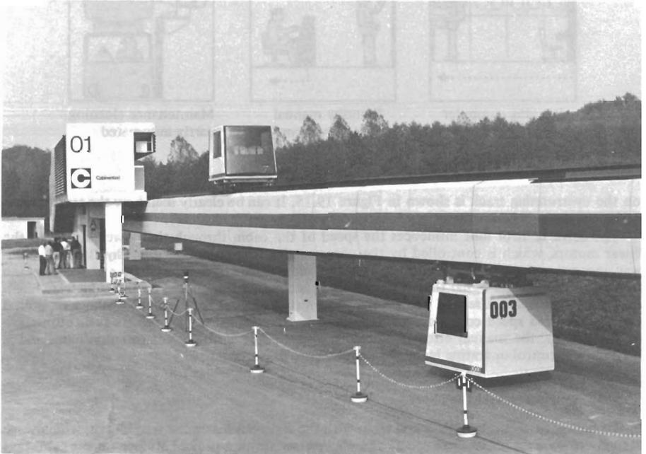
FIGURE 19.14 First construction phase of the trial circuit with station 01 and small-capacity cabs.
