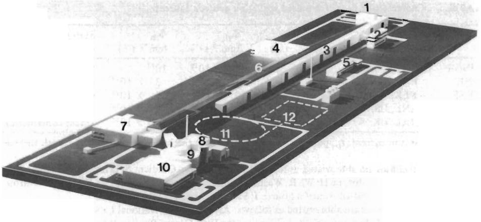
FIGURE 4 A model view of the SNQ facility. The buildings of the basic concept are shown together with the locations foreseen for the compressor ring and a future pulsed neutron source: 1, injector building; 2, test buildings; 3, RF gallery; 4, 350-MeV experimental area; 5, operations building; 6, accelerator tunnel; 7, 1100-MeV experimental area; 8, maintenance building; 9, target building; 10, neutron-guide hall; 11, future compressor ring; 12, future pulsed source.
