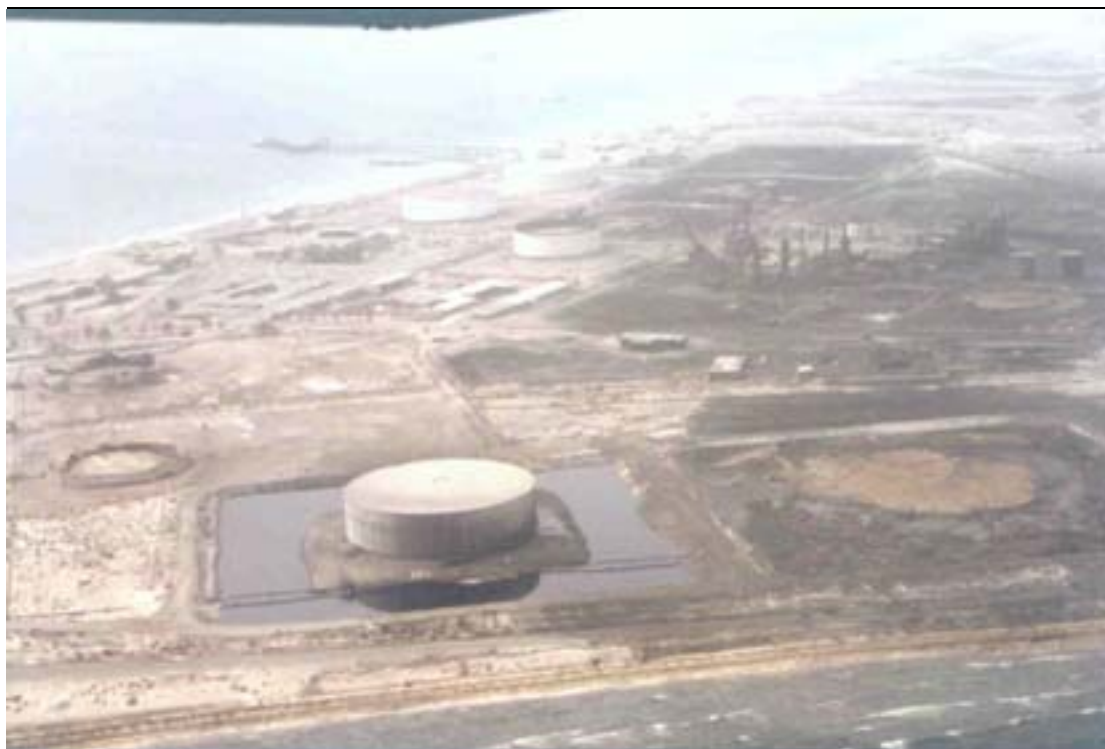
Figures 11 and 12. Exploded oil installations at the Al-Ahmadi Refinery, April 1991
